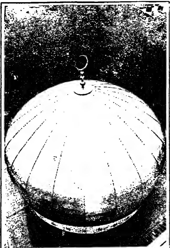
MOSQUE DOME -- The gold-coloured dome of the new $4 million Central Mosque stands out against the backdrop of trees in London's Regents Park. Its timber frame is sheathed in copper anodised with a gold finish and is protected by British architect Sir Frederick Gibberd and built by John Laing Construction Ltd.
